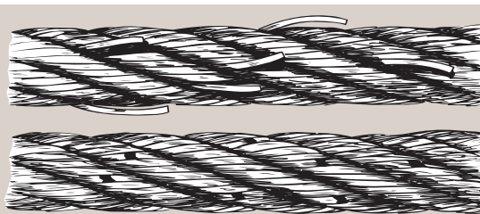
Typical valley (above) and crown (below) wire breaks in outer wires.
